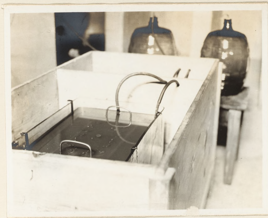
Fig. 26. Part of the respiration chamber devised by Galeotti in Naples.
