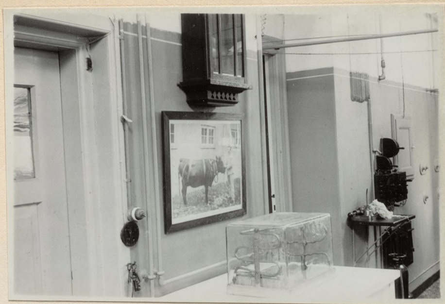
Figure 59 . Copenhagen, Denmark. Agricultural Experiment Station, Department of Physiology, Laboratory of Professor Møllgaard. Rabbit chamber showing glass cover and cooling pipes.
